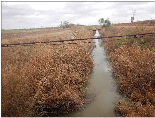
Photograph 37 – View looking northeast (downstream) at the existing Delta Lake Drain from the FM 490 bridge.
