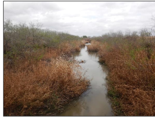
Photograph 40 – View looking north (downstream) at the existing Delta Lake Drain from CR 2900 West.
