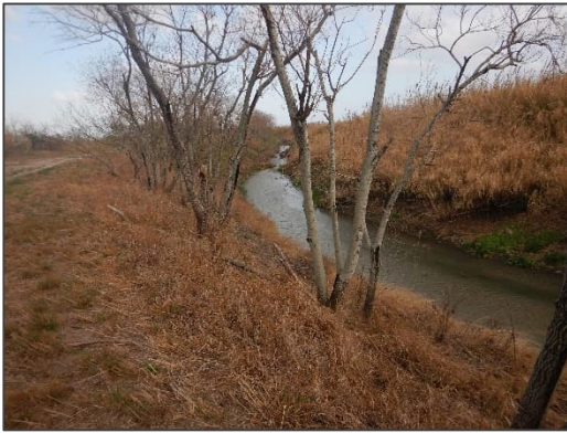
Photograph 25 – View looking east at the existing Delta Lake Drain, east of the location depicted in the previous photograph.
