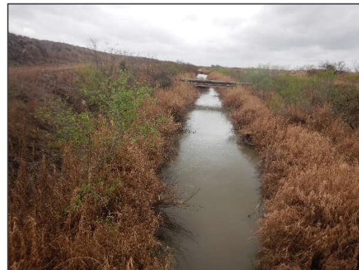
Photograph 36 – View looking southwest (upstream) at the existing Delta Lake Drain from the FM 490 bridge.
