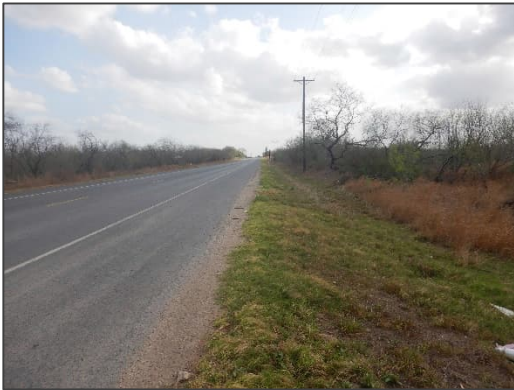
Photograph 13 – View looking south at FM 493. The existing Delta Lake Drain flows west to east under FM 493 via a box culvert.
