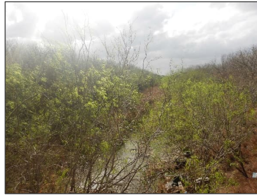
Photograph 10 – View looking west (upstream) at the existing Delta Lake Drain from Private Culvert Crossing #4.
