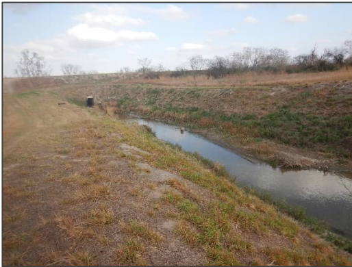
Photograph 19 – View looking east (downstream) at the existing Delta Lake Drain as it flows beneath the Delta Lake Irrigation Channel (higher in elevation than the RDP).
