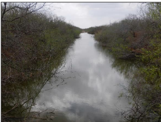
Photograph 2 – View looking west at the existing Delta Lake Drain from Private Culvert Crossing #1.
