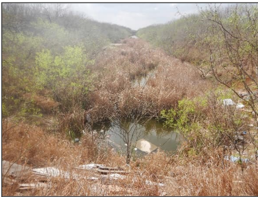
Photograph 8 – View looking west (upstream) at the existing Delta Lake Drain from Private Culvert Crossing #3.
