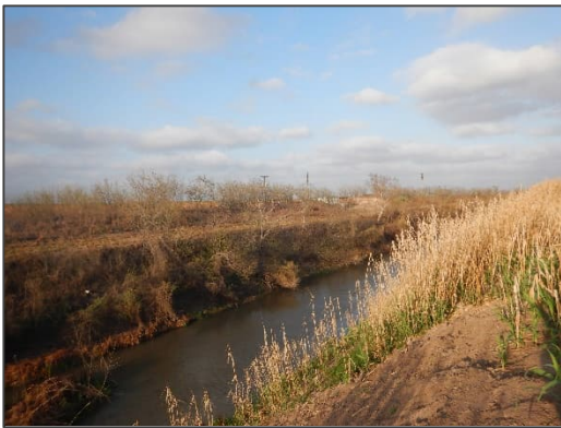
Photograph 26 – View looking northeast (downstream) at the existing Delta Lake Drain where it is adjacent to Delta Lake. Delta Lake is separated from the existing Delta Lake Drain by an access road and maintenance berm.
