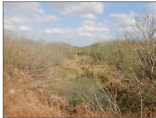
Photograph 11 – View looking east (downstream) at the existing Delta Lake Drain from Private Culvert Crossing #4.
