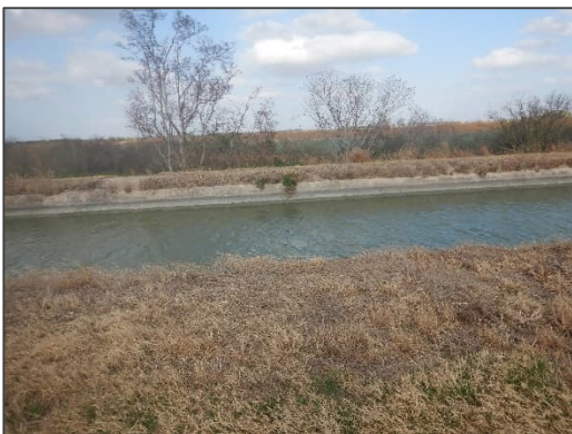
Photograph 21 – View looking northeast at the Delta Lake Irrigation Channel, which flows through a structure over the existing Delta Lake Drain.
