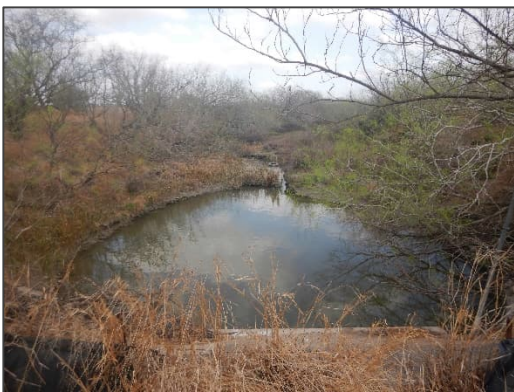
Photograph 14 – View looking east (downstream) at the existing Delta Lake Drain from the FM 493 bridge.
